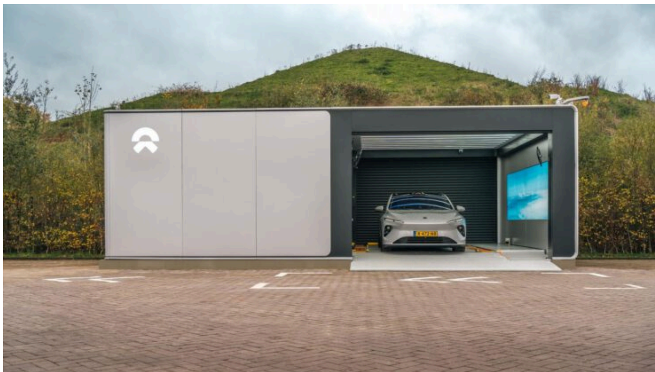
Power Swap Station Hotel Tilburg
